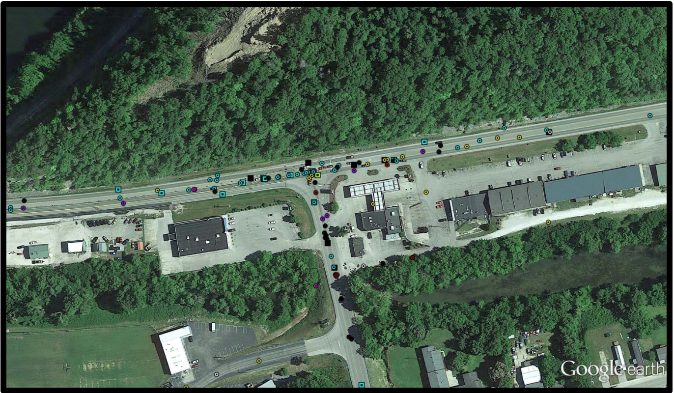
Intersection #2 KY 15 (MP 17.446) at Washington Avenue
