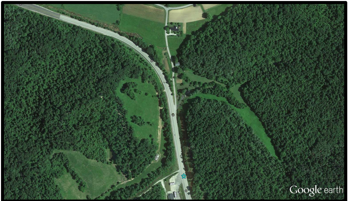
Intersection #39 KY 15 (MP 8.235) at Swift Camp Road
