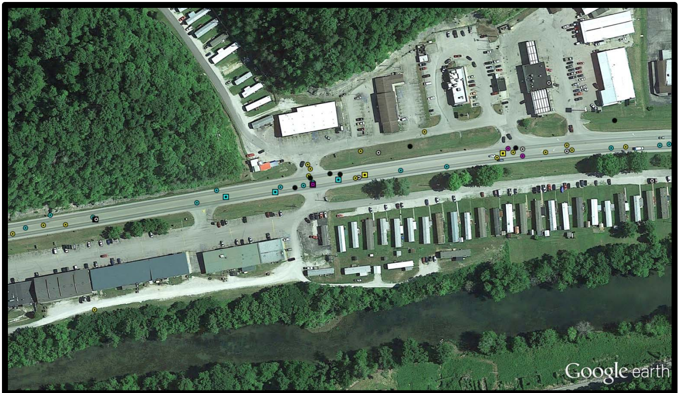
Intersection #8 KY 15 (MP 17.253) at Indian Hollow Road
